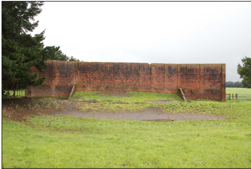
The butt of the 25-yard rifle range at Featherston Camp, built in 1918 ( Bargas & Shoebridge/MCH )
