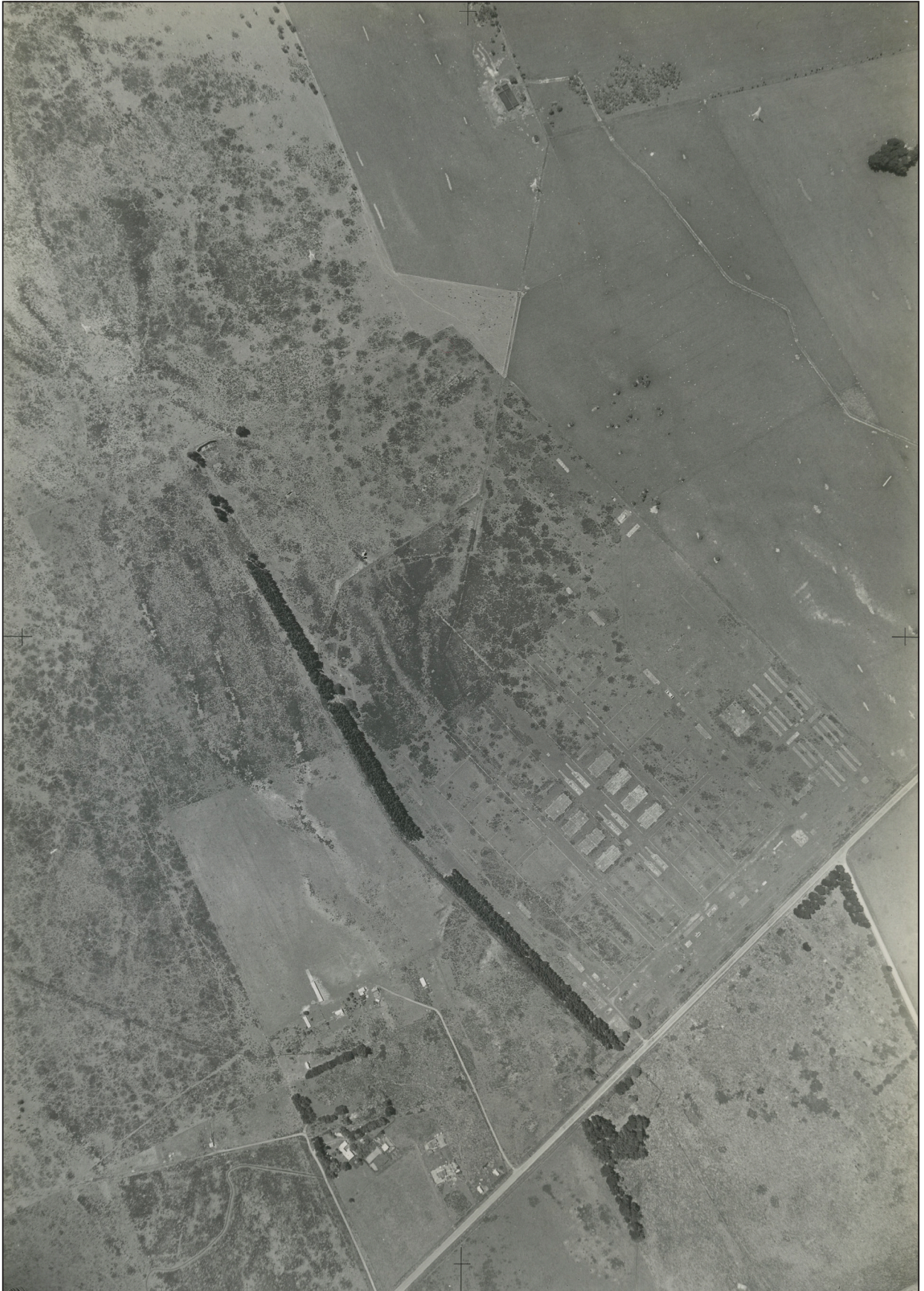
The site of Featherston Camp in November 1941, less than a year before the Japanese prisoner of war camp was built on the site. The camp's water-race filter-bed is visible in the top-centre of the photo. (AALJ W3492 2, Archives NZ)
