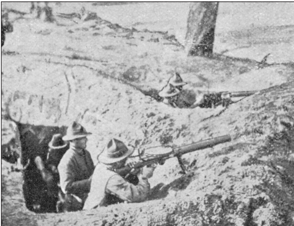
The machine gun emplacements at Papawai Camp, c1917 ( Stanbrook )
